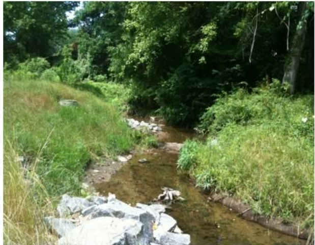
Figure 4-8: Stabilized stream banks
