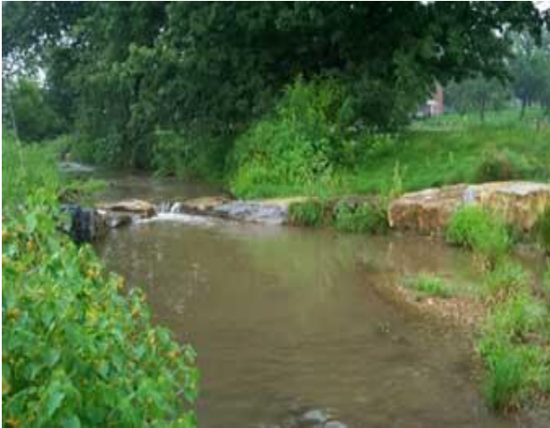
Figure 4-7: Cross vane added to stream
