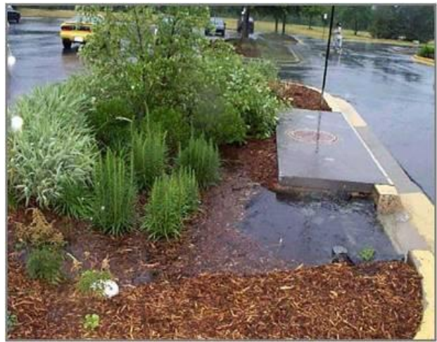
Figure 4-4: Parking lot bioretention filter
