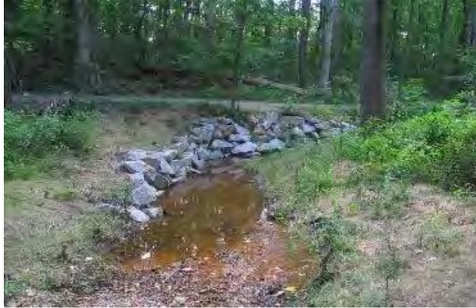
**Figure 4: Typical riprap bank protection (VA DEQ)**
