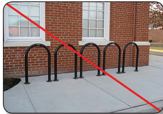
Incorrect positioning of Inverted "U" Racks
