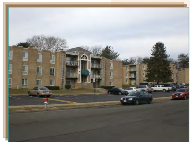
Adjacent Merrifield at Dunn Loring Station apartment complex
