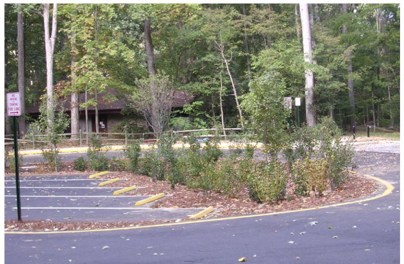
Figure 38: Rain Garden in Parking Lot Example
